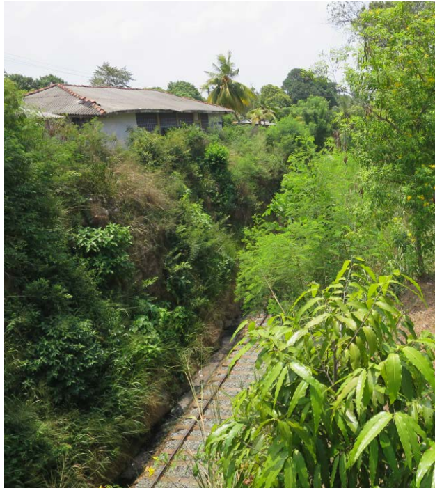
Figure 3-8: Existing line deeply excavated near Kesbewa road, just after Nugegoda station
